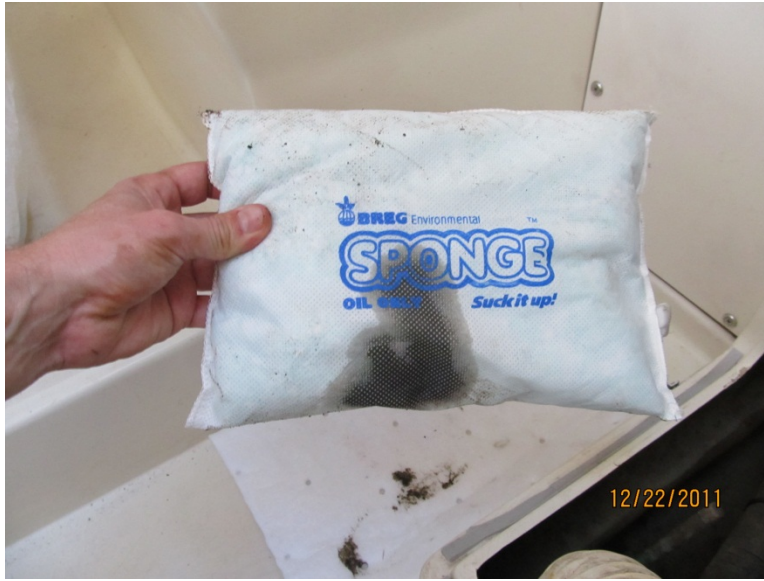
Figure : Oil absorbent pillow wedged between oil pan and engine bed captured any oil bypassing the pads.
